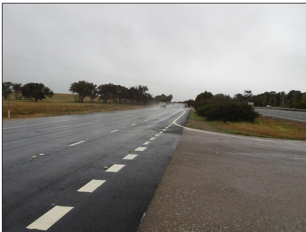
Figure 3A: Federal Highway Facing East from near the Quarry
