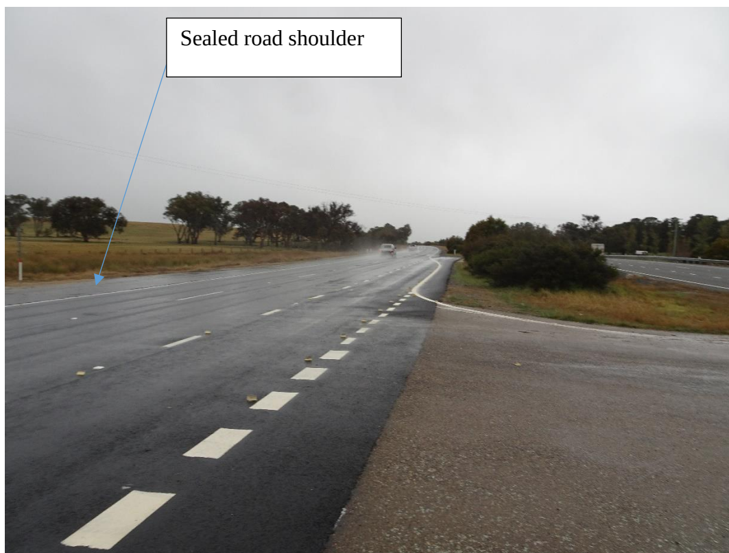
Figure 3B: Federal Highway Facing East from near the Quarry showing sealed road shoulder
